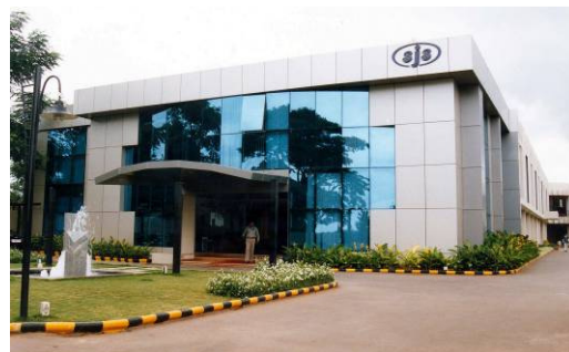
Photo 5. SJS Enterprises' prestigious purpose-built office and factory on the outskirts of Bangalore, India.
